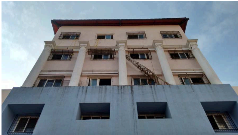
Figure 19. Postmodern back façade comprising of five columns
