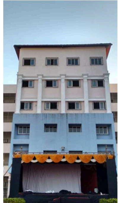
Figure 20. Postmodern back façade comprising of five columns
