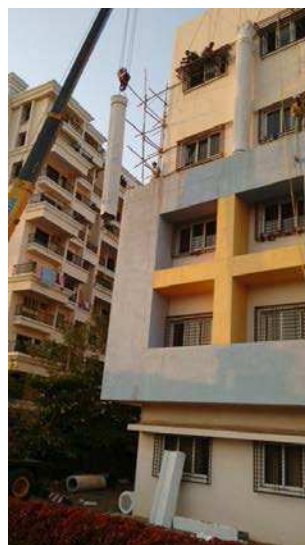
Figure 18. Erected with a crane
