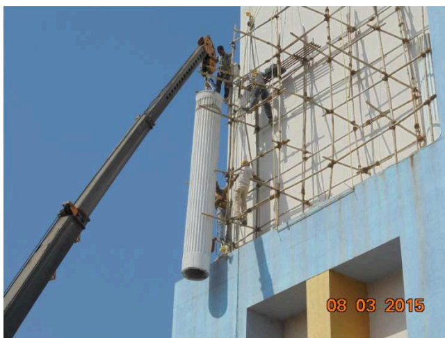
Figure 17. Erected with a crane
