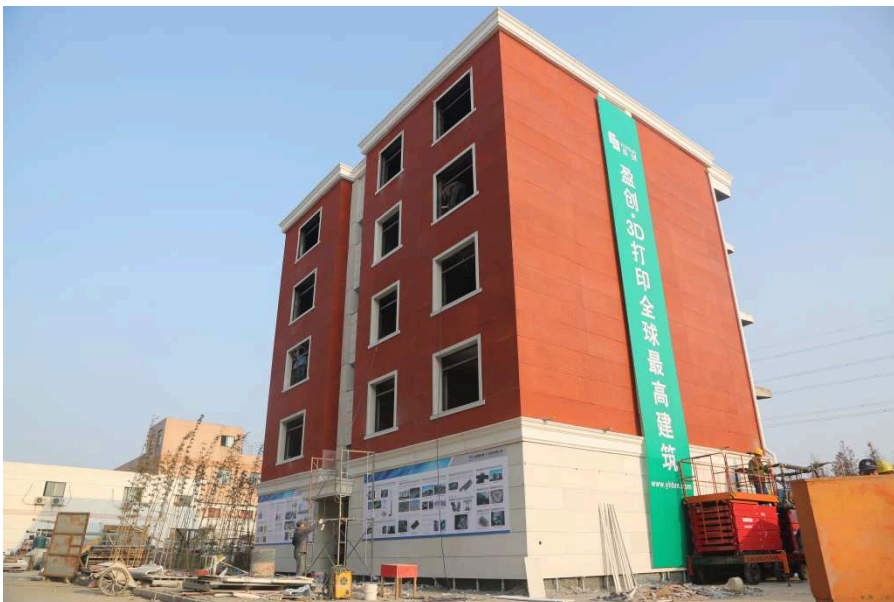
Figure 7. 3D printed 6-story building
