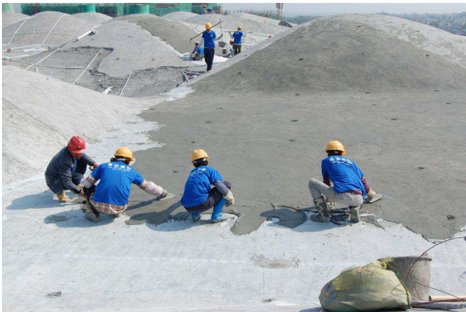
Figure 3. Insulation layer construction
