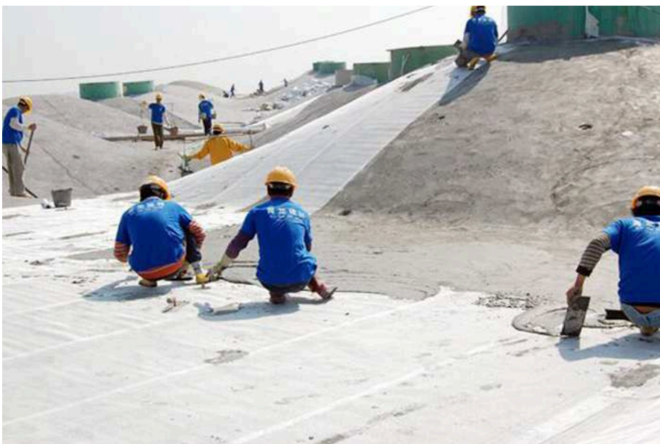
Figure 6. Applying fiberglass mesh
