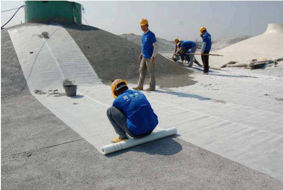
Figure 5. Applying fiberglass mesh
