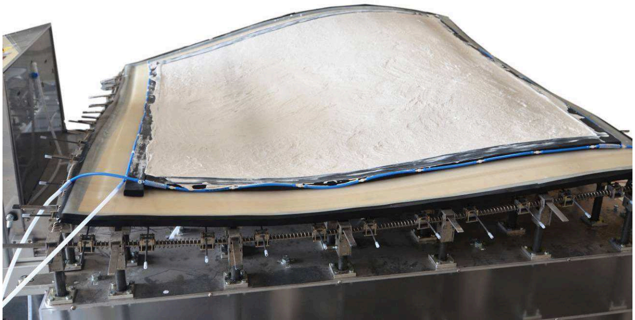
Figure 2. Casting of a double curved fiber reinforced concrete panel ( www.adapa.dk ).
