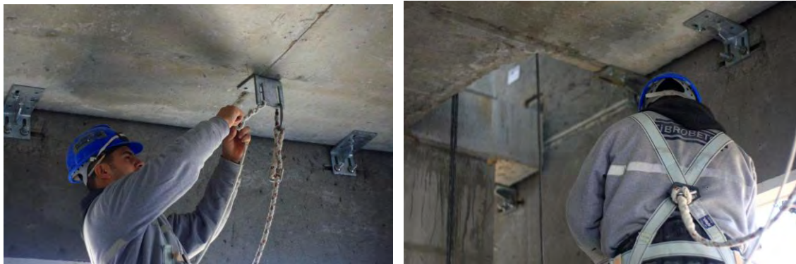
Figure 3. An appearance from actual installation of wall panels
