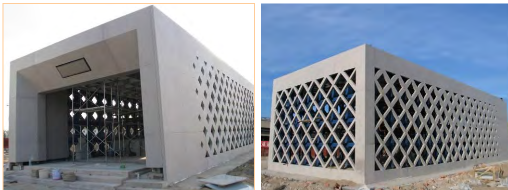
Figure 12 Entrance of subway station
