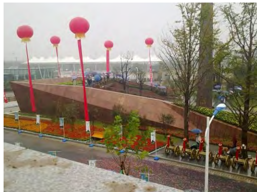
Figure 14 Army Exhibiting Hall in Zhengzhou Virescence Exposition
