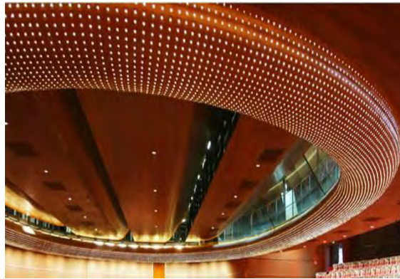
Figure 4 GRC in the opera house of the National Grand Theatre
