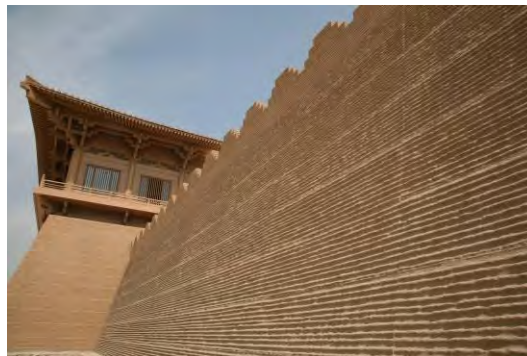
Figure 5 Hybrid panels of GRC and concrete in Xi'an Daming Palace
