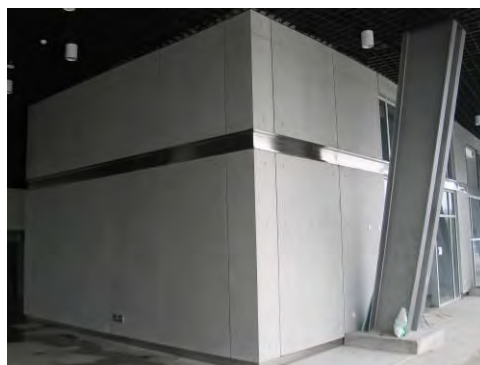
Figure 10 GRC panel used in elevator rooms in the National Olympic Athletics Centre
