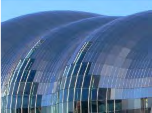
Figure 7: The open-joint system with waterproof layer below on the Sage Music Center in Gateshead,
