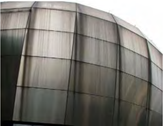
Figure 7: The open-joint system with waterproof layer below on the Sage Music Center in Gateshead,
