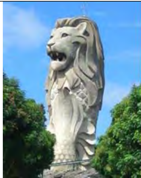
FIGURE 10: 37m High Singapore's National Icon; The Merlion, Sentosa Island; GRC Free Form Structure
