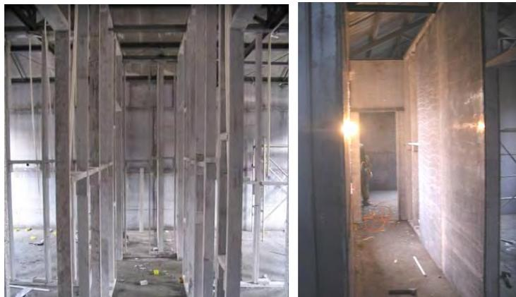
**Figure 8 Installation of partition wall**
