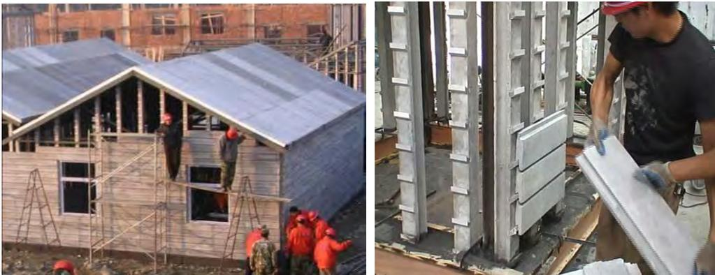
**Figure 6 Installation of cladding panels and finished view**
