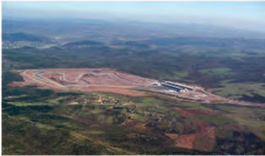
Figure 1 - Photo of construction of Formula 1 track
