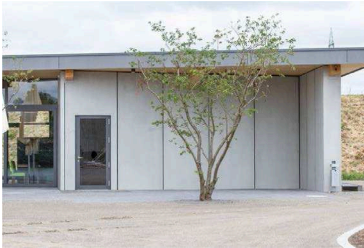
Figure 6: Ventiladed curtain wall (SchieferErlebnis, Dormettingen)
