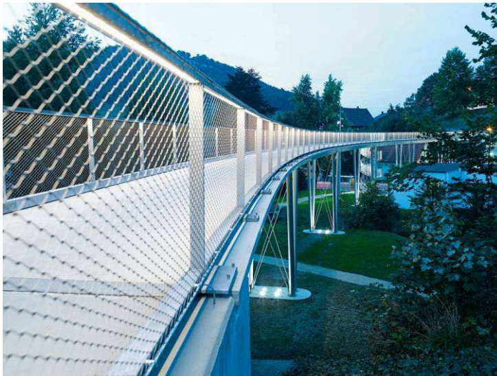
Figure 9: Pedestrian overpass in Albstadt
