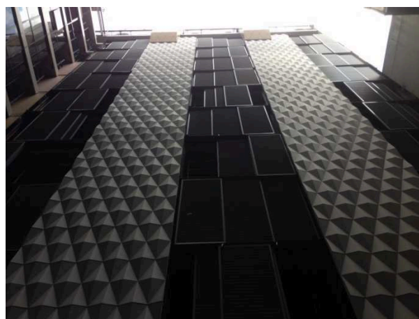
Figure 5. Flinders Street – Offices, Melbourne (2013)
