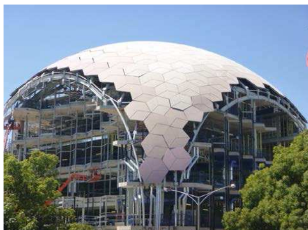
Figure 17. Asurco - Geelong Library, Geelong (in progress)
