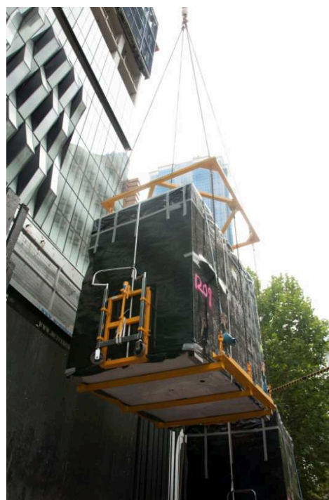
Figure 14. Bathroom Floor – Complete module being craned into building
