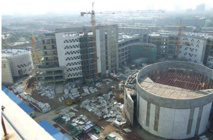
Fig.2 The construction site of the Huhhot Youth Centre
