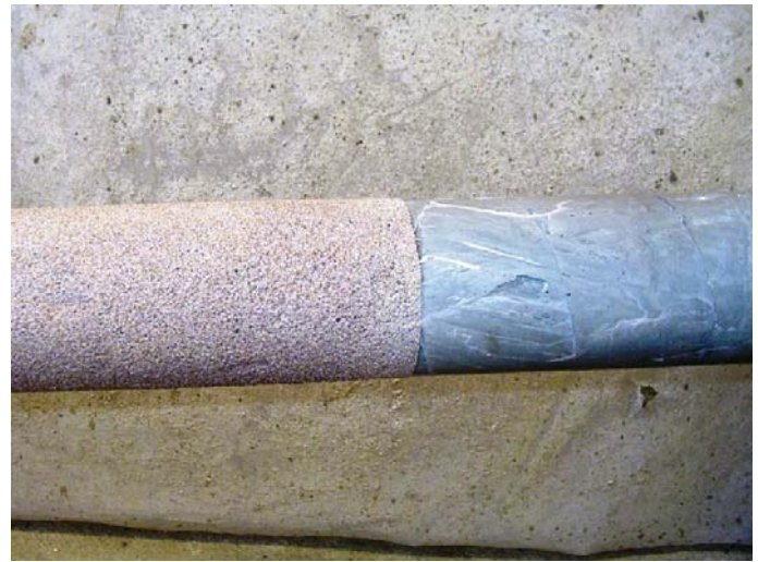
Figure 4: Sprayed mortar finishing
